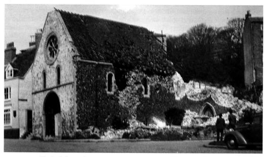
Fig. 7. St James, Dover, 9 May 1950, after collapse of war-damaged tower. Ministry of Works (English Heritage, NMR)
